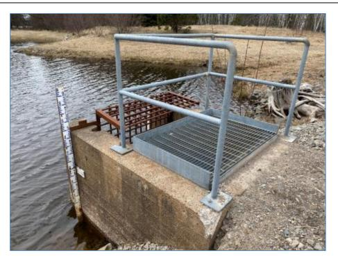
Figure 18-58: Discharge Weir
