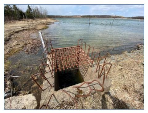
Figure 18-48: Tailings Storage Facility Decant Tower
