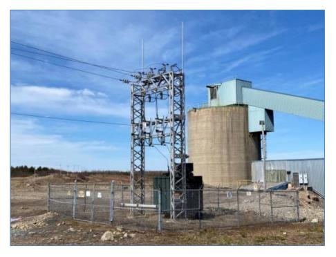
Figure 18-4: 8,000 kVA Transformer
